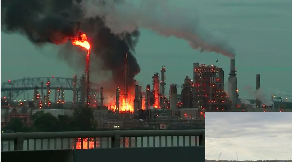
PES Refinery Explosion, South Philadelphia ( CNN )
